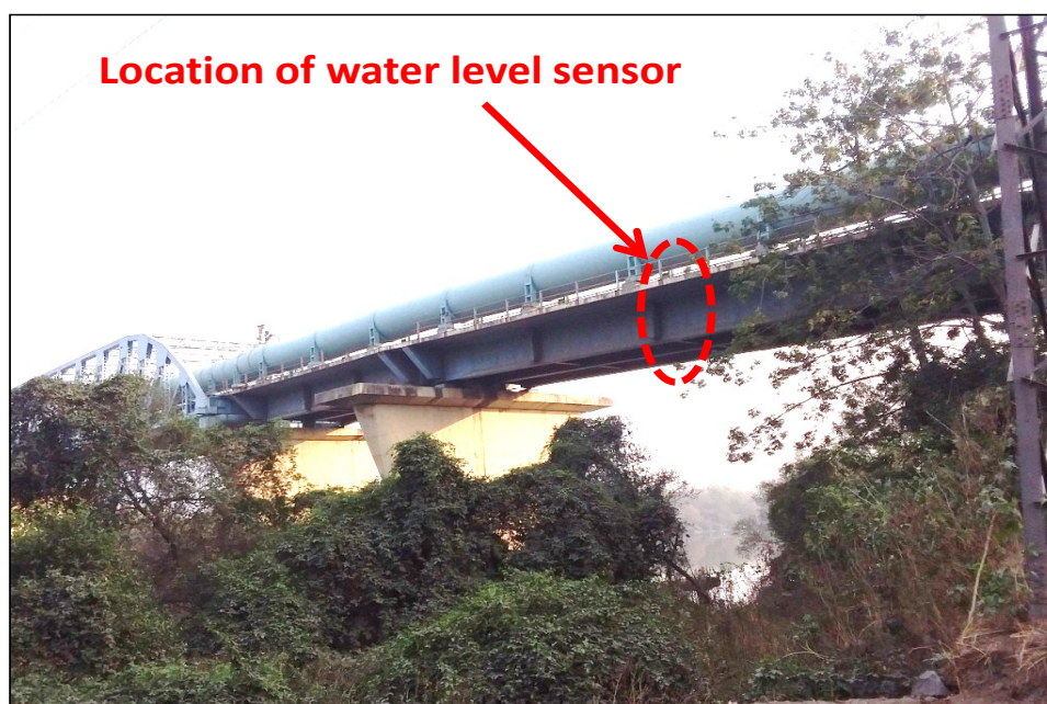
Figure 2. Location of real-time water levels sensors on Saket pipe line bridge
